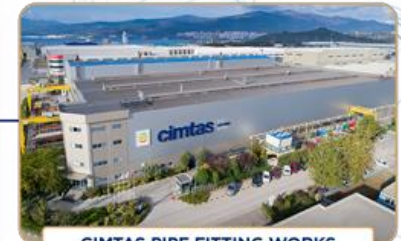
ÇİMTAŞ PIPE FITTING WORKS
